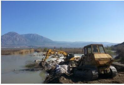
At the Kargi hydropower plant in Turkey a study to measure the potential benefits of increased water efficiency downstream of the dam on the Kizilirmak River was initiated in 2016. The overall goal is to verify if there is potential for reducing water released and increasing generation.
